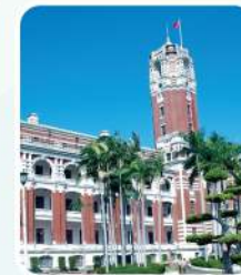
Presidential Office Building (Government)
